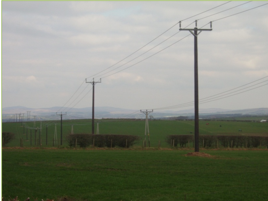
Figure 10-1: 33kV overhead line resilient rebuild of 'A' pole line (in background), SPD
