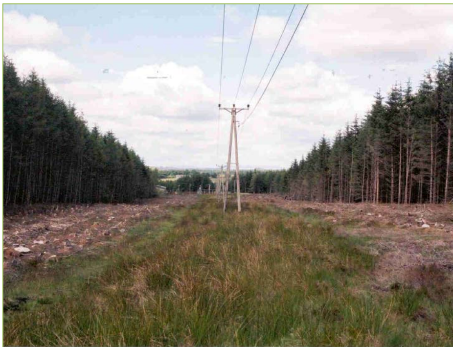
Figure 10-4: 33kV overhead line following tree clearance as part of our Rural Care programme, a precursor to ETR132
