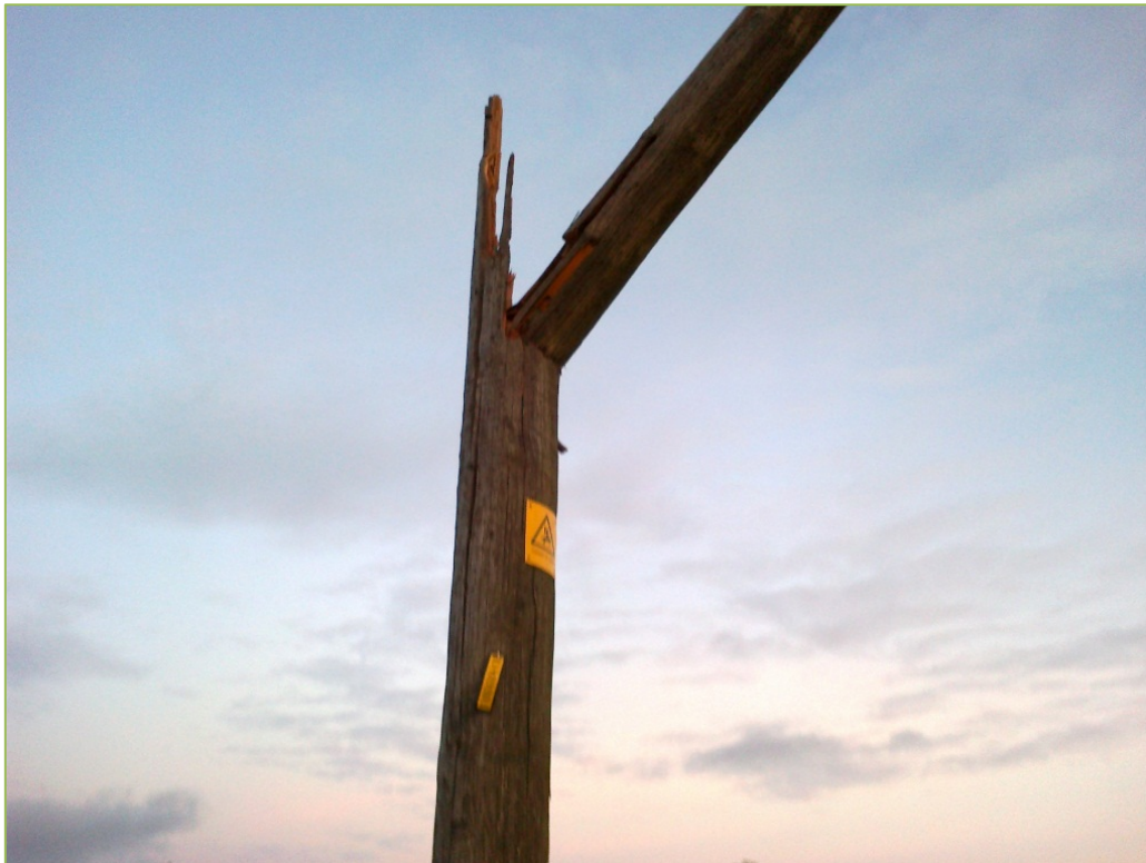
Figure 10-6: Example of pole damage following severe weather
