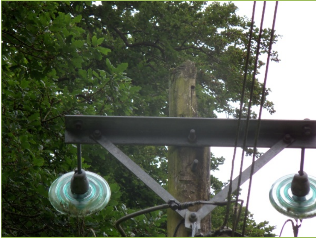
Figure 10-5: Example of pole top rot
