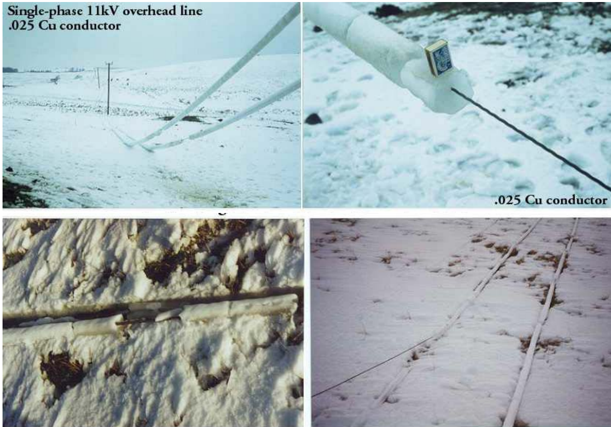
Figure 10-7: Examples of faults due to ice accretion on overhead line conductors during storm events on non-resilient lines, SPD
