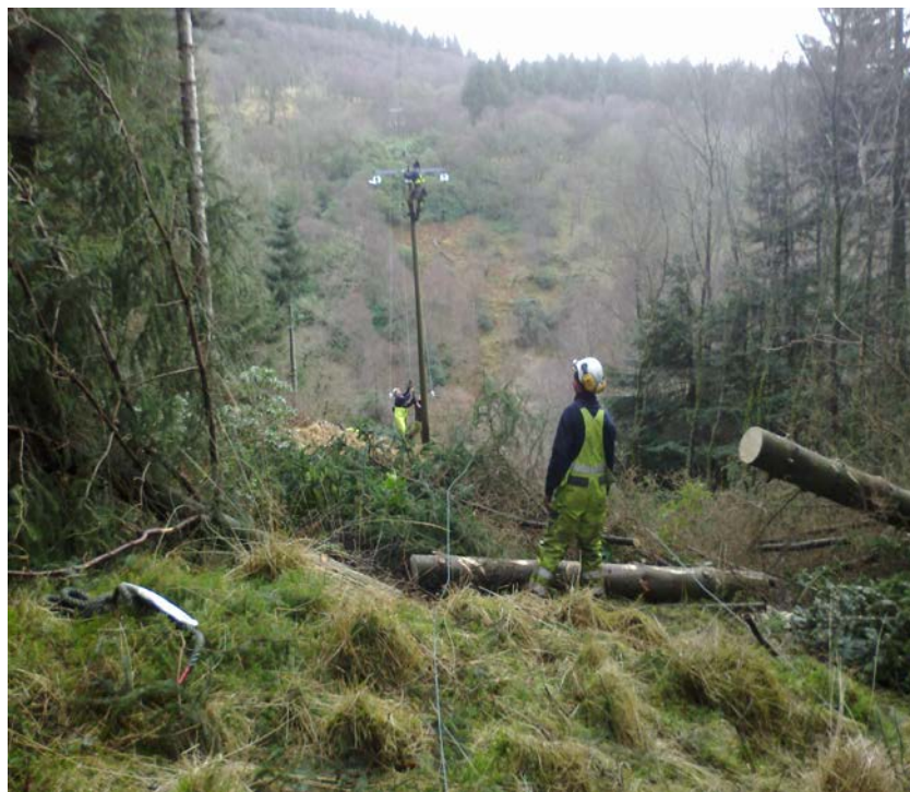
Figure 10-2: Repairing damage caused by falling trees, January 2012 storm, SPD
