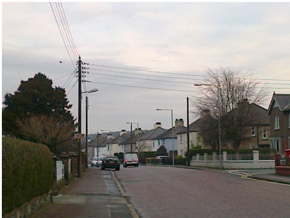
Figure 8-2: LV overhead lines prior to Village Modernisation, SPD
