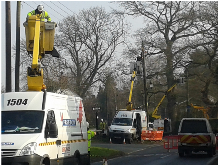
Figure 8-1: LV Village Modernisation works underway, SPM
