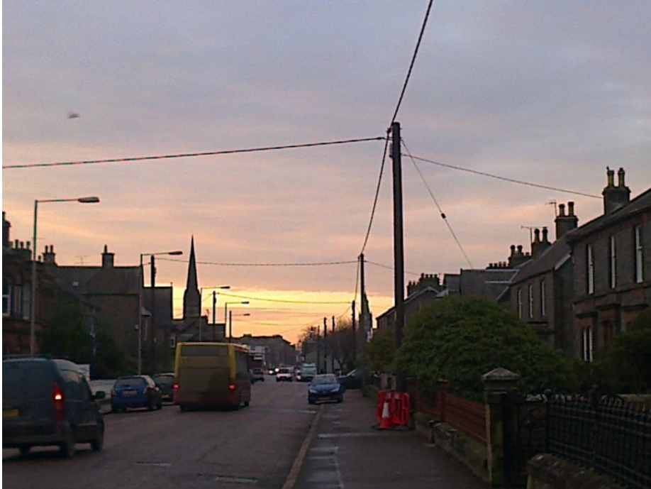
Figure 8-3: LV overhead lines following Village Modernisation, SPD
