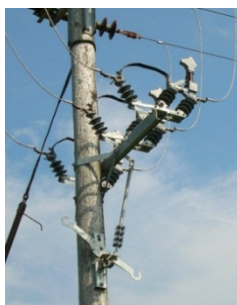
Pole mounted switch
