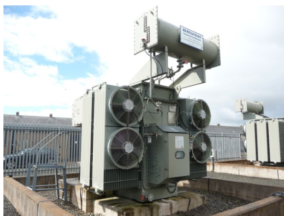
New banded transformer
