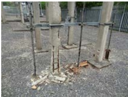
Substation support structure
