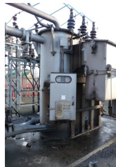
33kV transformer
