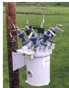
Pole mounted circuit breaker
