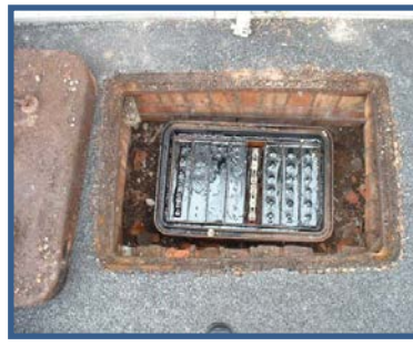
LV underground link box
