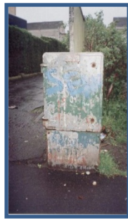
LV street pillar
