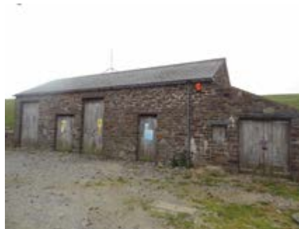
Primary substation building
