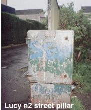
showing excessive corrosion and bungs missing
