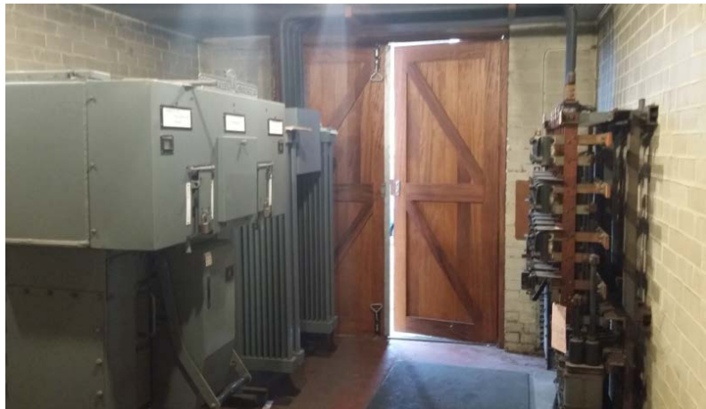
Figure A6: A typical Y-Type 11/0.430kV non unit protected substation the SPM network
