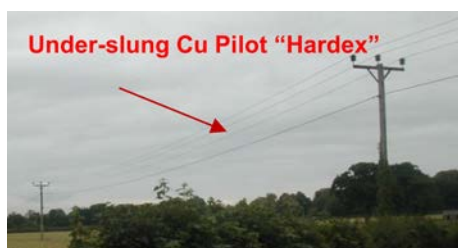
Figure 6: Hardex on a 33kV Overhead Line
