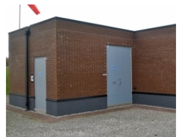
Tulip Primary substation
