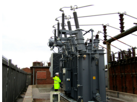
Speke Grid replacement
