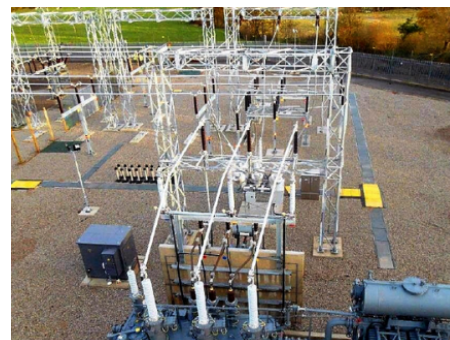
St Asaph Grid new transformer
