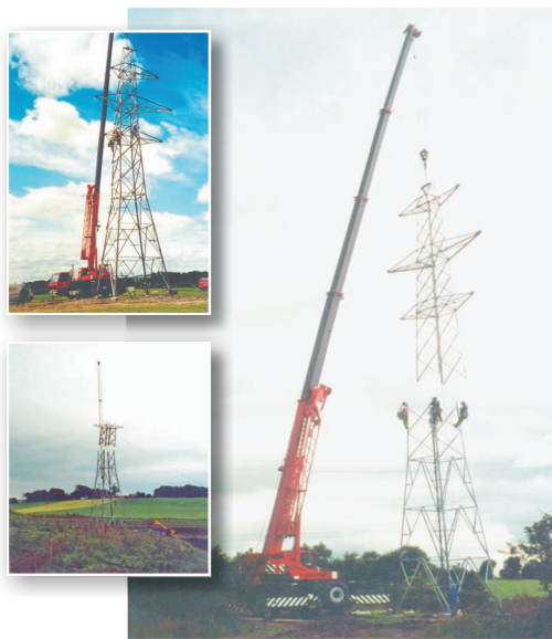
Construction of typical L4 tower
