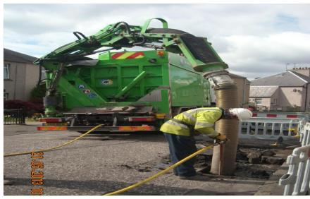
The above image demonstrates the advantages of new technology where a vacuum excavator is being utilised to remove spoil from the excavation by suction with the aid of an air lance.
