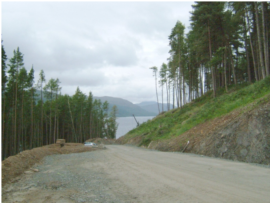
Plate 1: Cut Track in Rock (Note provision of passing place. Drainage ditch still to be installed at foot of cut)
