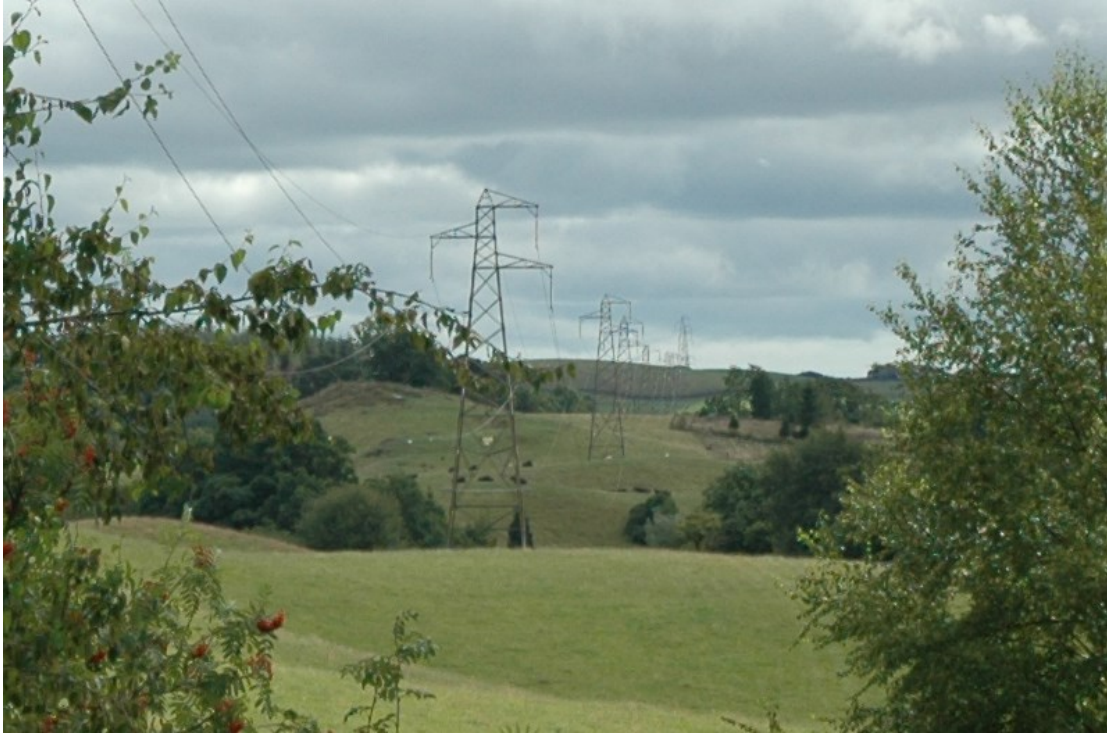
Figure 3: The single circuit 132kV transmission overhead line between Glenlee and Tongland
