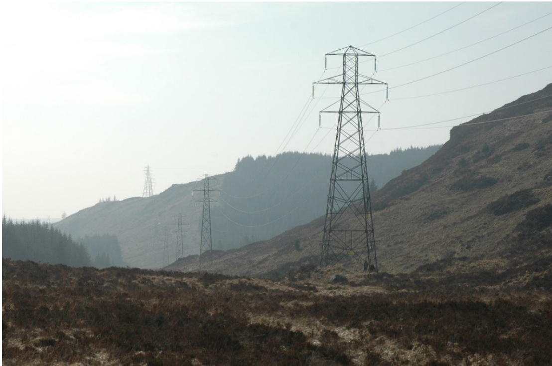
Figure 2: The double circuit 132kV transmission overhead line between Newton Stewart and Glenlee
