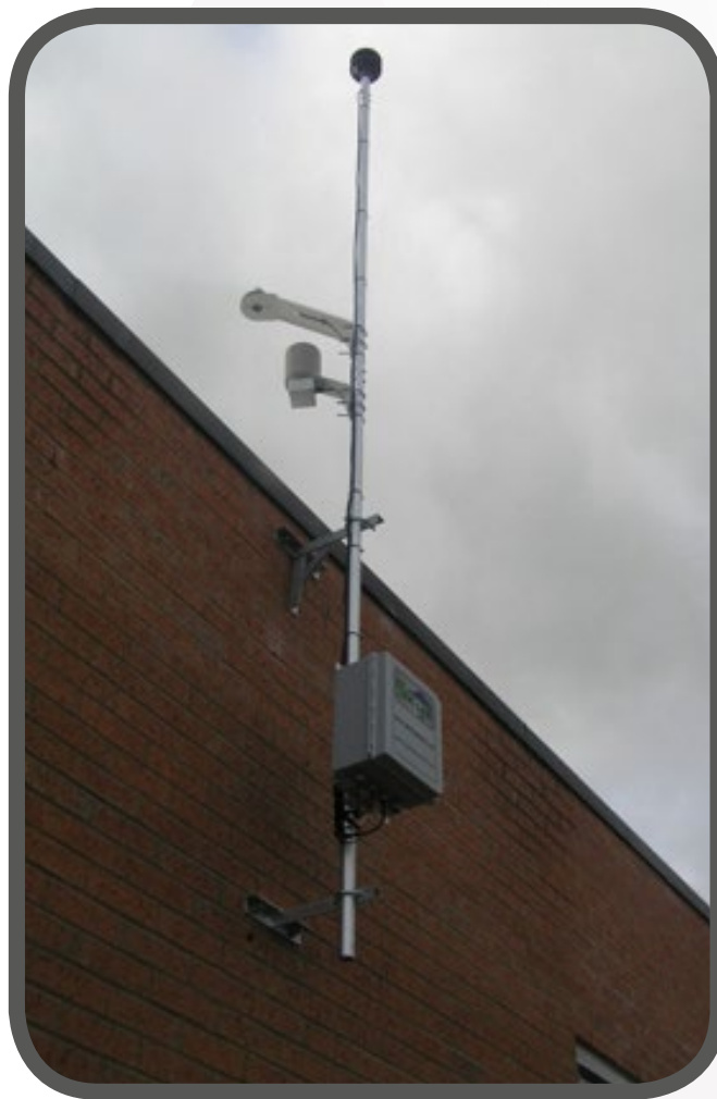
Figure 9: Building-mounted RTTR monitoring equipment installed at a substation
