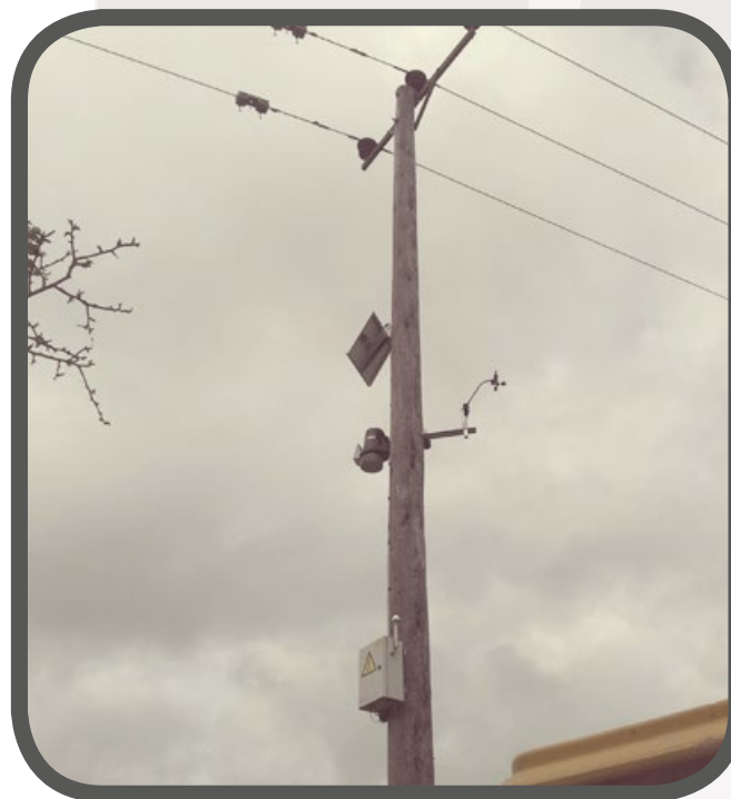
Figure 11 RTTR monitoring equipment installed on a 33 kV pole
