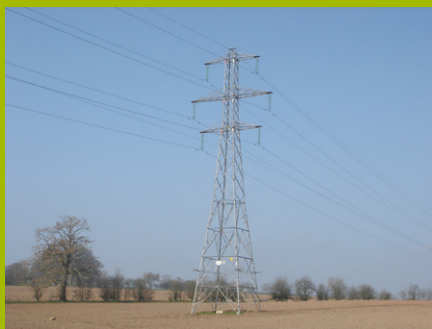
L7 (C) Lattice Tower (double circuit arrangement).
