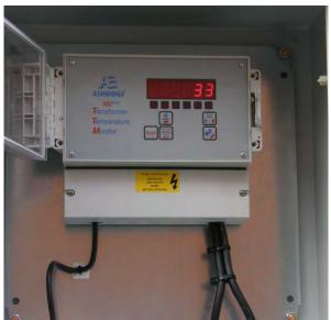
The 852plus is an electronic unit and using an electrical PT100 sensing probe which fitted into the existing temperature probe pocket replacing the existing WTI capilliary probe. The transducer output signal to the substation monitor was connected via a dedicated twisted pair cable.
