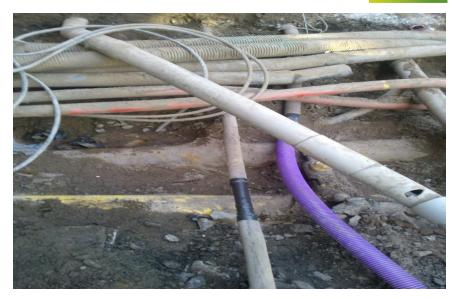
The above image highlights an incident where an operative removed the lead sheathing from a ScottishPower EnergyNetworks 0.3(4) main underground low voltage electrical cable.
