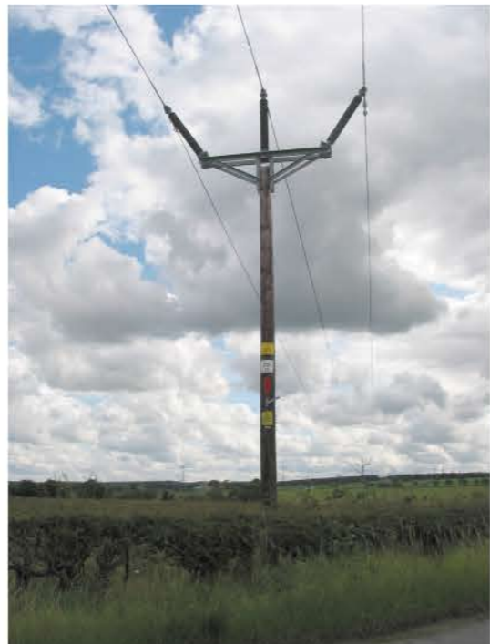
Trident single pole, 'trident' insulators
