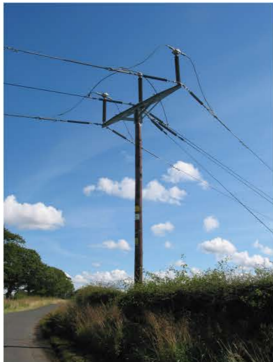
Trident single pole, vertical insulators
