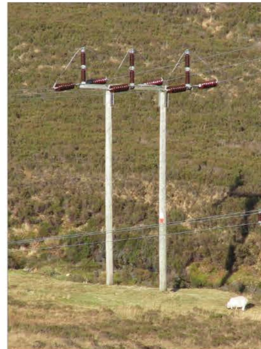
Trident 'H' pole straight-line pole
