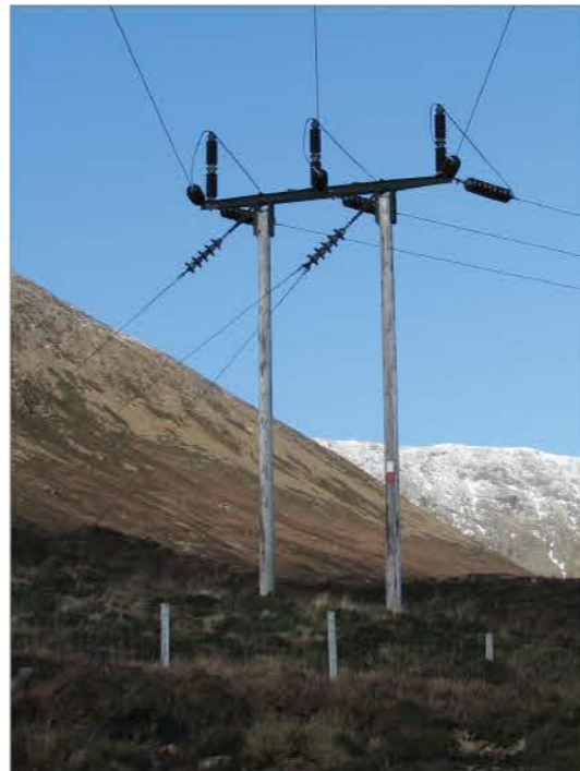
Trident 'H' pole turning pole
