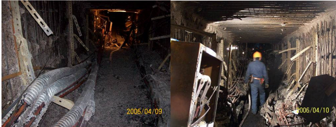
Figure 1 - Fire Damage in a Cable Tunnel in China
