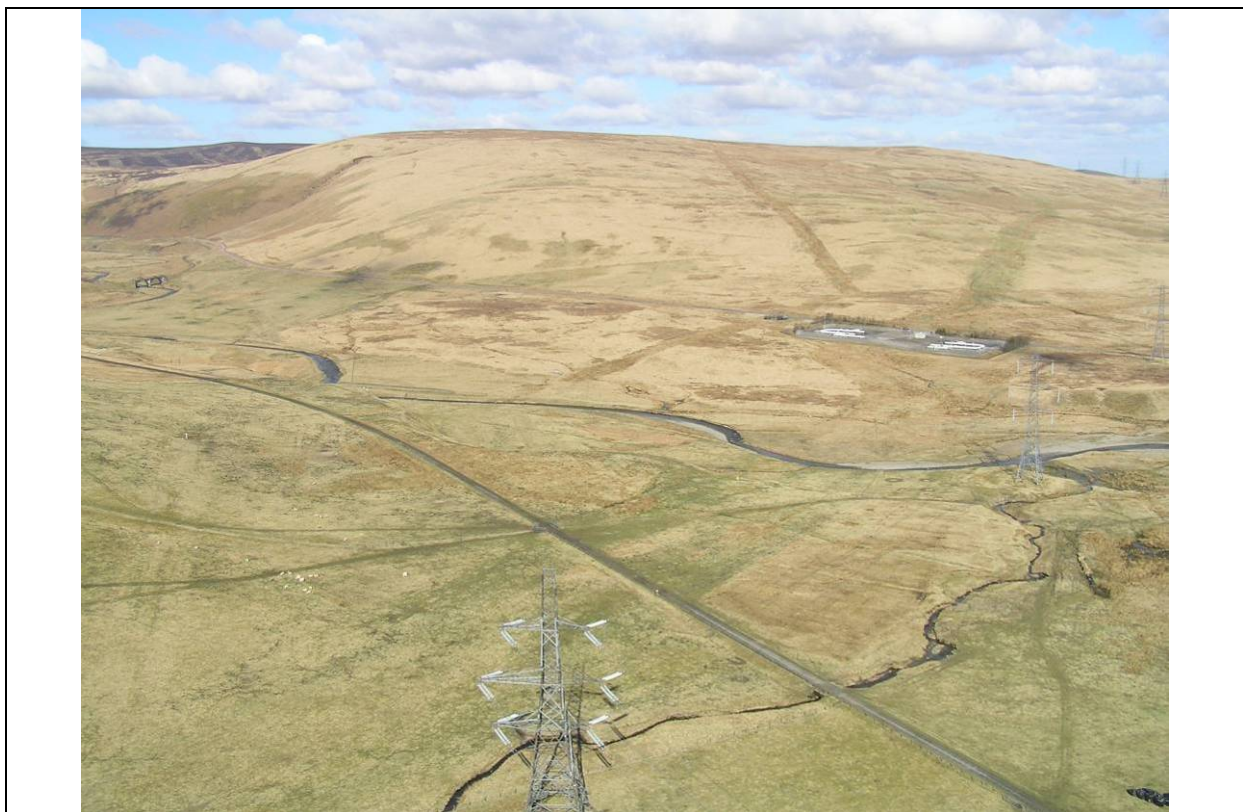
Figure 3-5 Gas pipelines visible from the air at Elvanfoot
