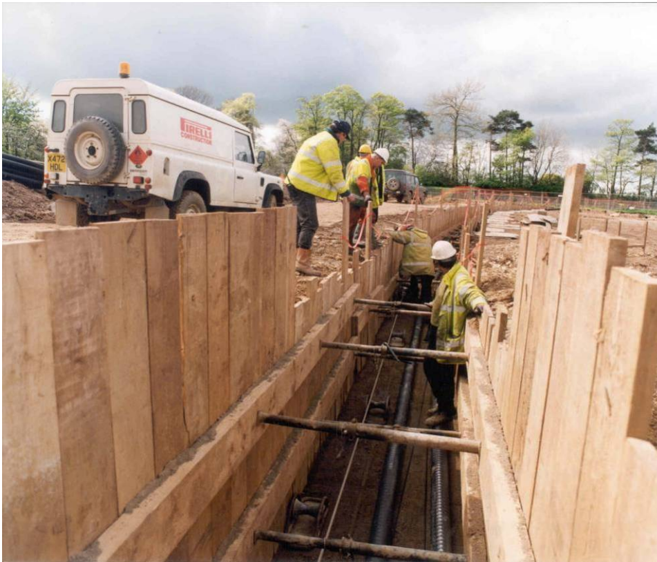
Figure 2-13 Cable installation in an open cut trench
