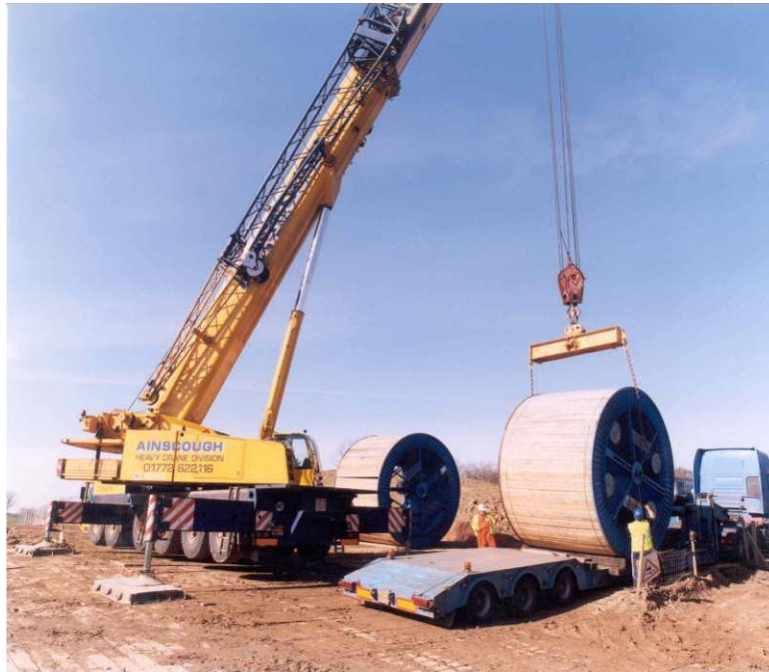
Figure 2-12 Offloading cable drums
