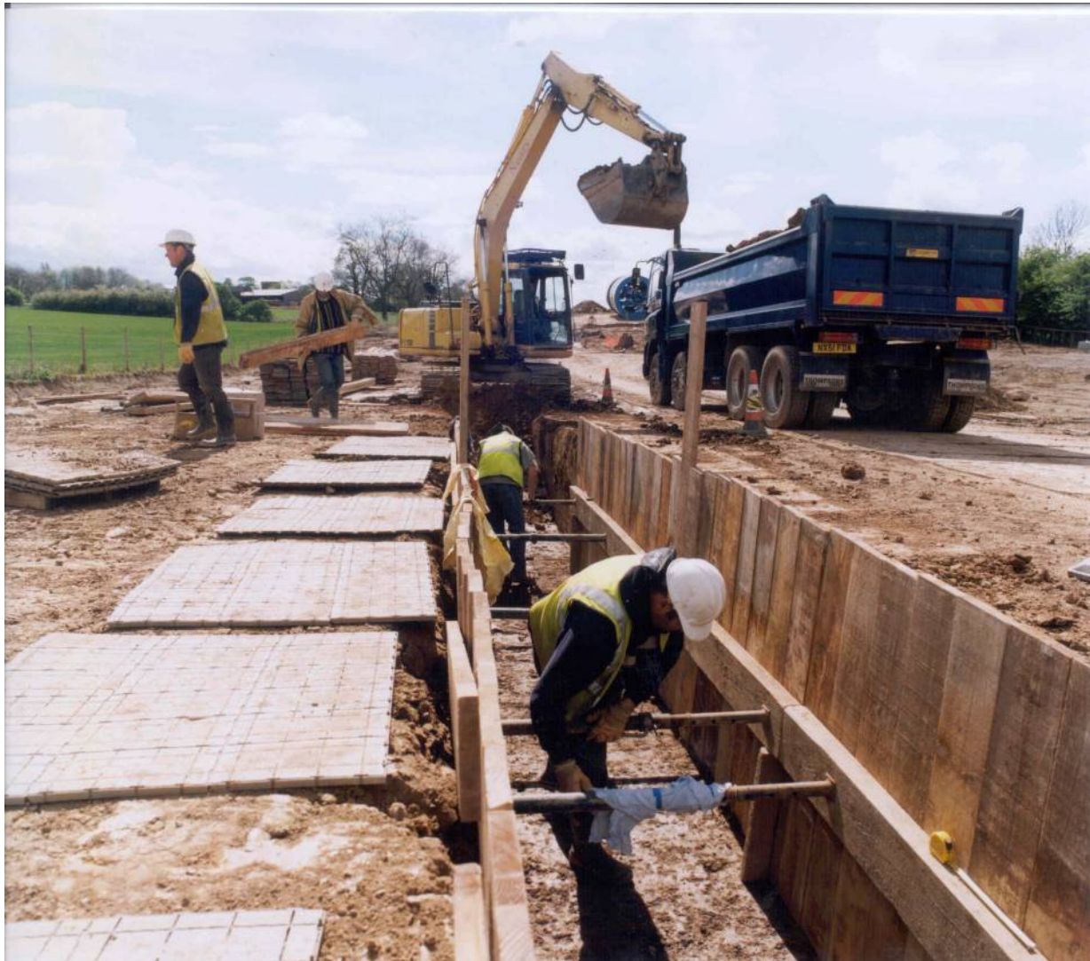
Figure 2-9 A close timbered cable trench
