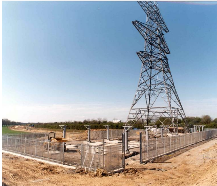
Figure 3-7 Overhead Line Cable Sealing End Compound Construction
