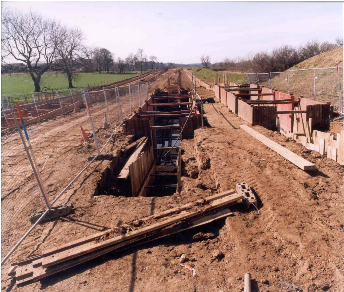
Figure 3-2 Excavation of a Joint Bay Position
