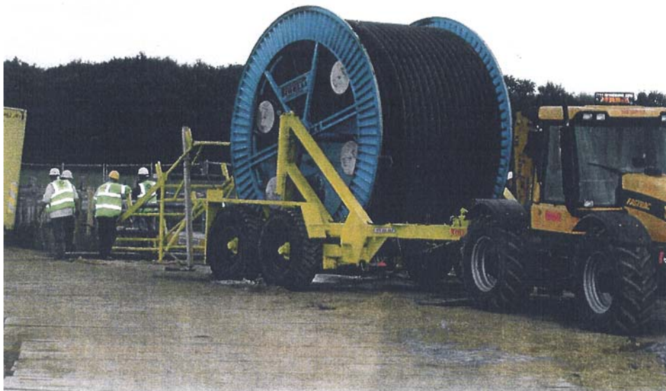
Cable drum and trailer
