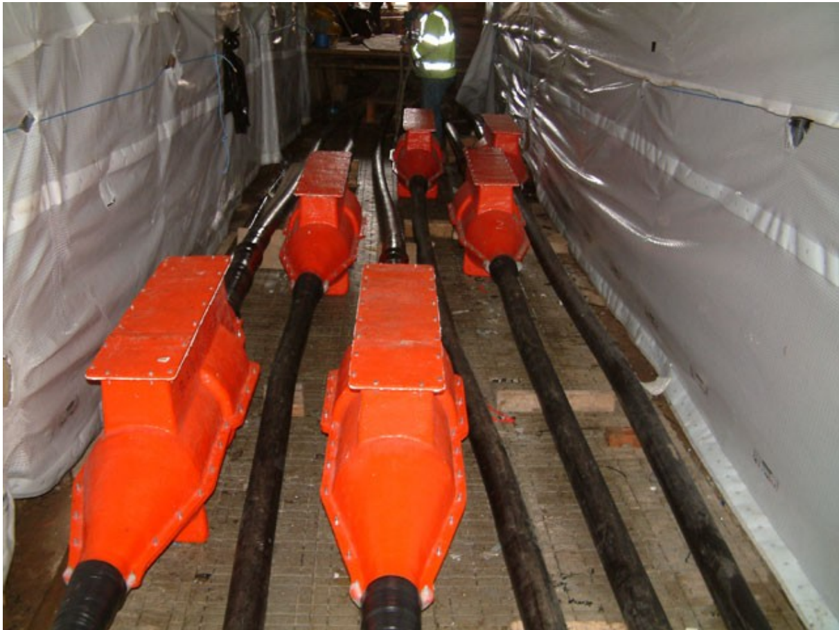
Figure 2-2 275kV Joint bay Containing Six Joints
