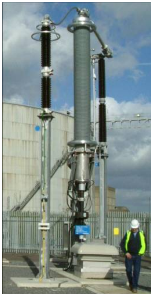
Figure 2-3 400kV Cable Outdoor Sealing End (ODSE) Termination
