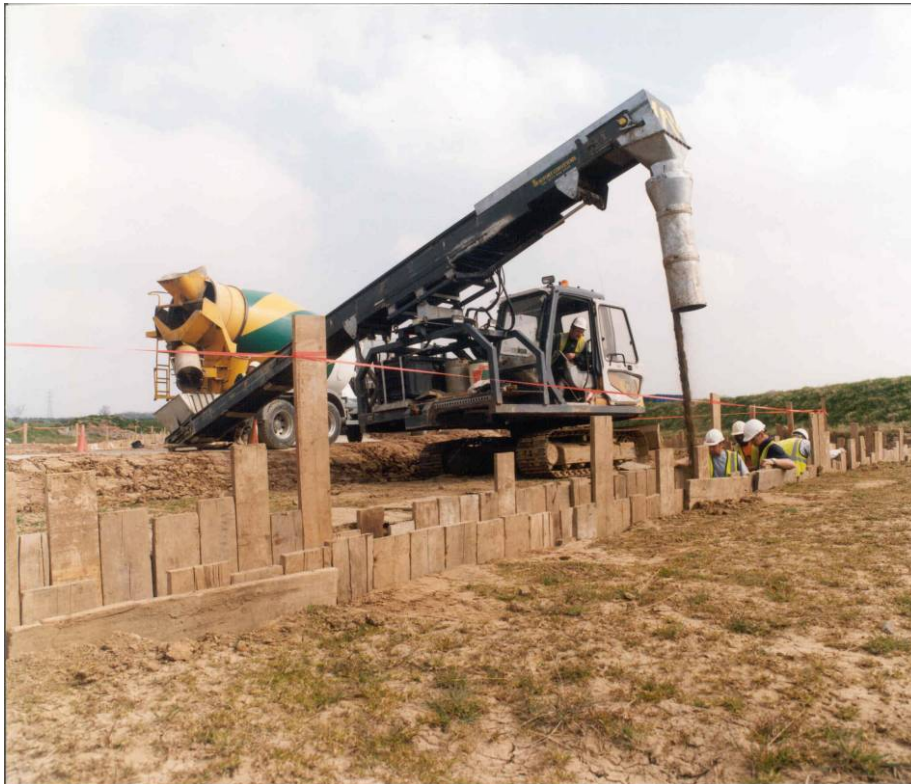
Figure 2-14 Delivery of CBS to the cable trench
