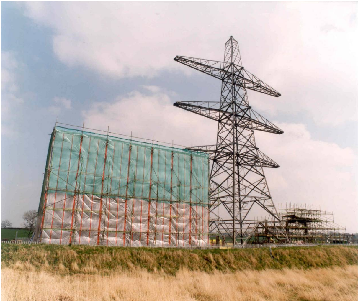
Figure 2-15 Weatherproof Sheeted Enclosure for Cable Termination Assembly
