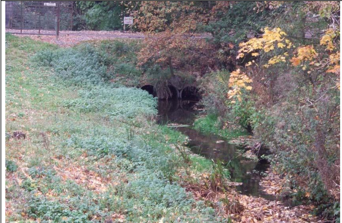
Figure 3-22: Water course alongside the A820 (as crossed by Nursery Access Road)
