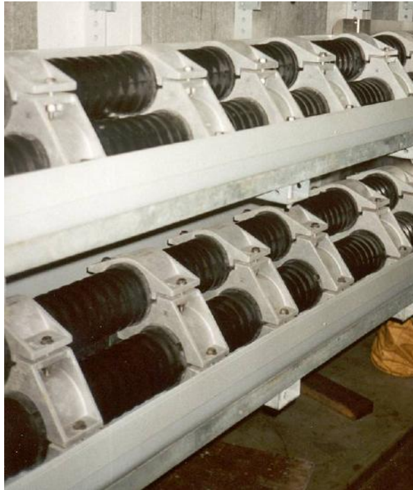
Figure 4-5: - EHV Cables Installed in Trefoil
