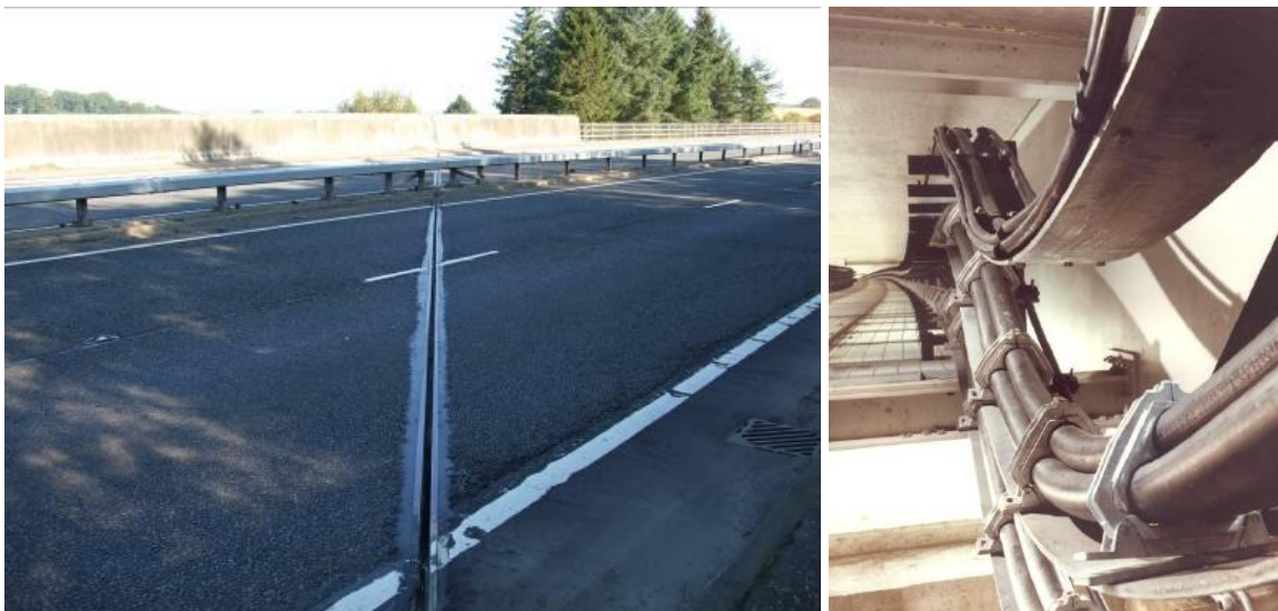
Figure 3-13: Expansion Joint and a Flexible Cable Crossing Design
