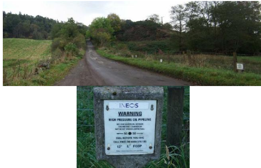
Figure 3-9: – Fuel Line Marker Posts at Bannock Burn Crossing
