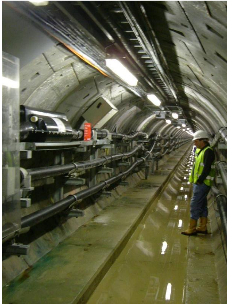
Figure 4-4: - 400kV Cable Joints and Phase Transposition
