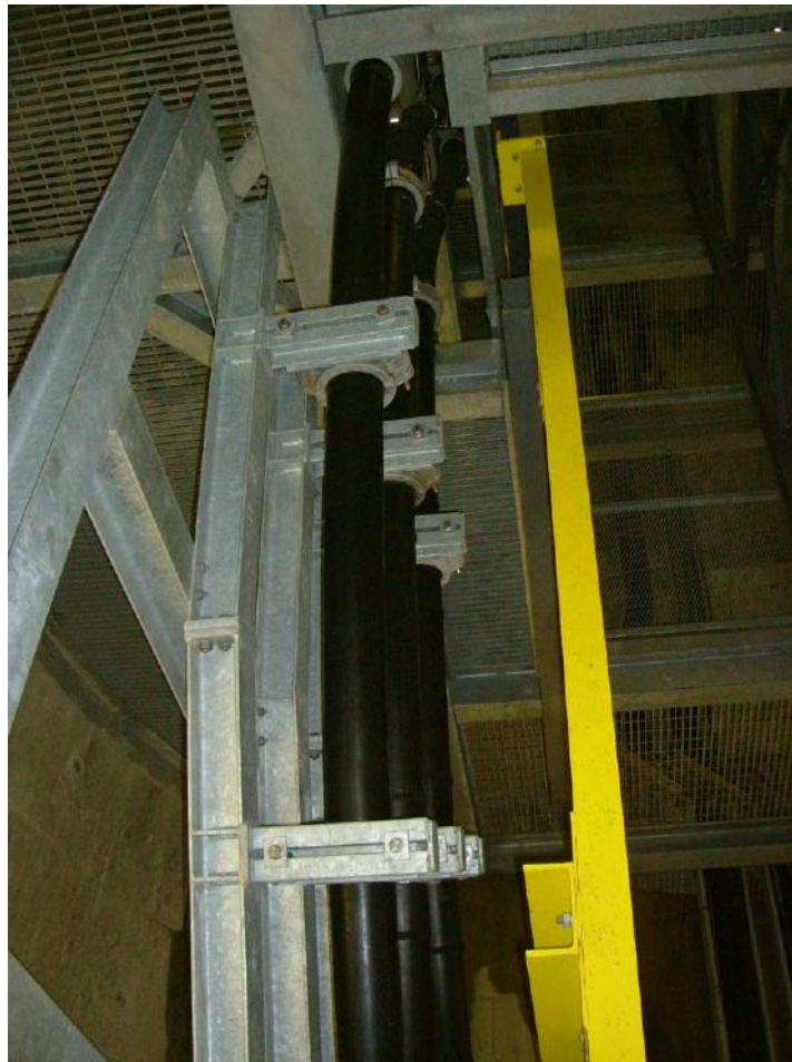
Figure 4-3: - 400kV Cables Cleated in a Tunnel Shaft
