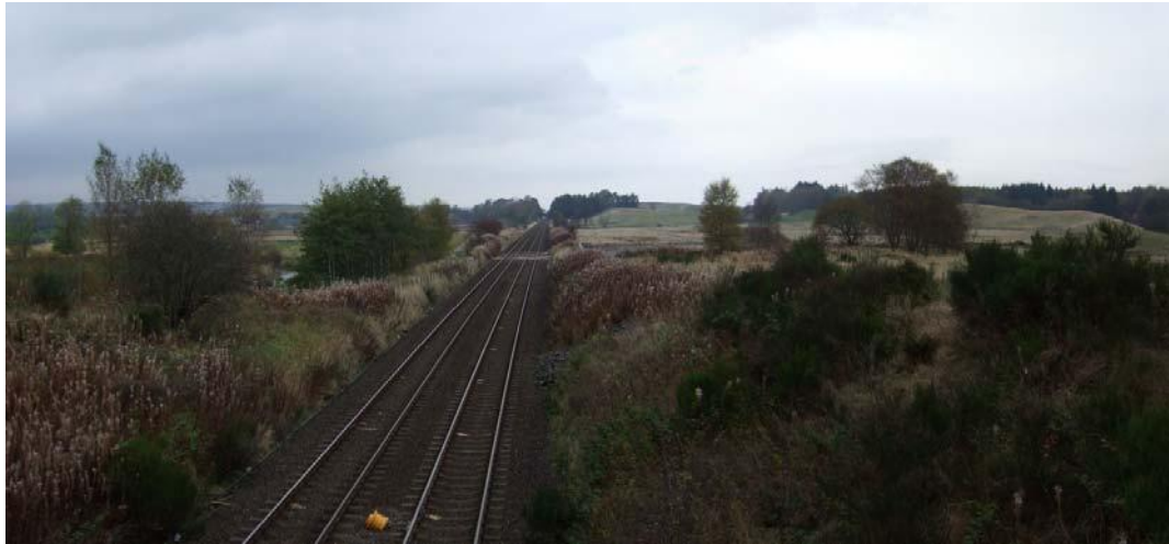
Figure 3-20: – Rail and Allan Water Crossing at Ashfield
