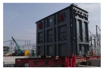
The majority of the work is now complete. The 300 tonne Transformer has been installed. The 275kv substation was energised in August 2014 and the 400kv substation energised November 2015. will continue through to the final completion mid-2016.
