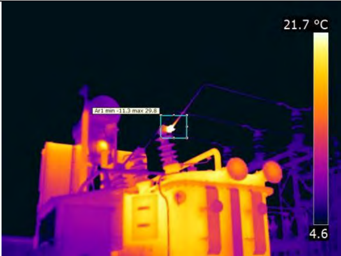
Hot spot on terminal of 33 kV-transformer bushing
