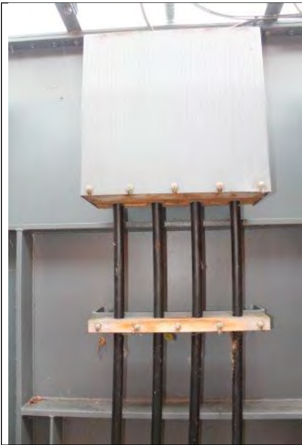
11 kV cable termination box, no signs for deterioration, ageing and leakage.
