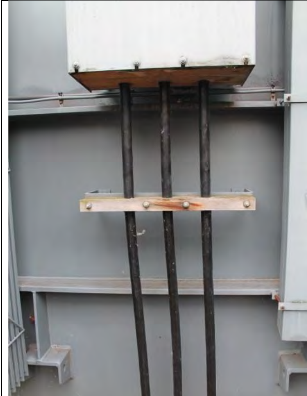
33 kV cable termination box, no signs for deterioration, ageing and leakage.
