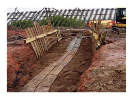
The above image demonstrates the size of excavations required to undertake the installation/repair of Transmission cables.
