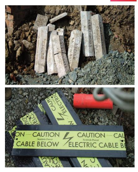
The above image demonstrates marker tiles utilized by SP Energy Networks to protect the Transmission cable network, the maker tiles should not be removed without consultation with ScottishPower.
