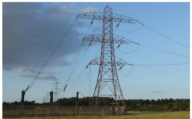
Terminal tower and cable sealing end platform
