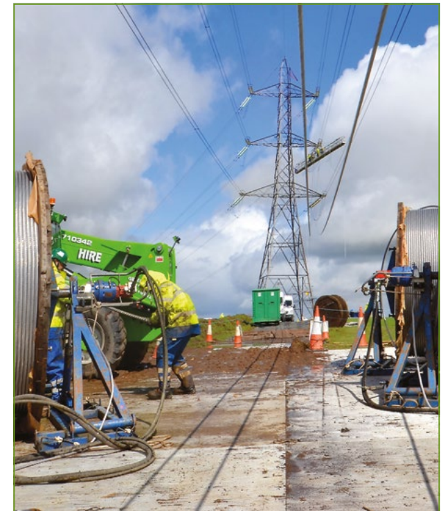
XV Route Overhead Line Modernisation – 72km delivered in 2013/14
