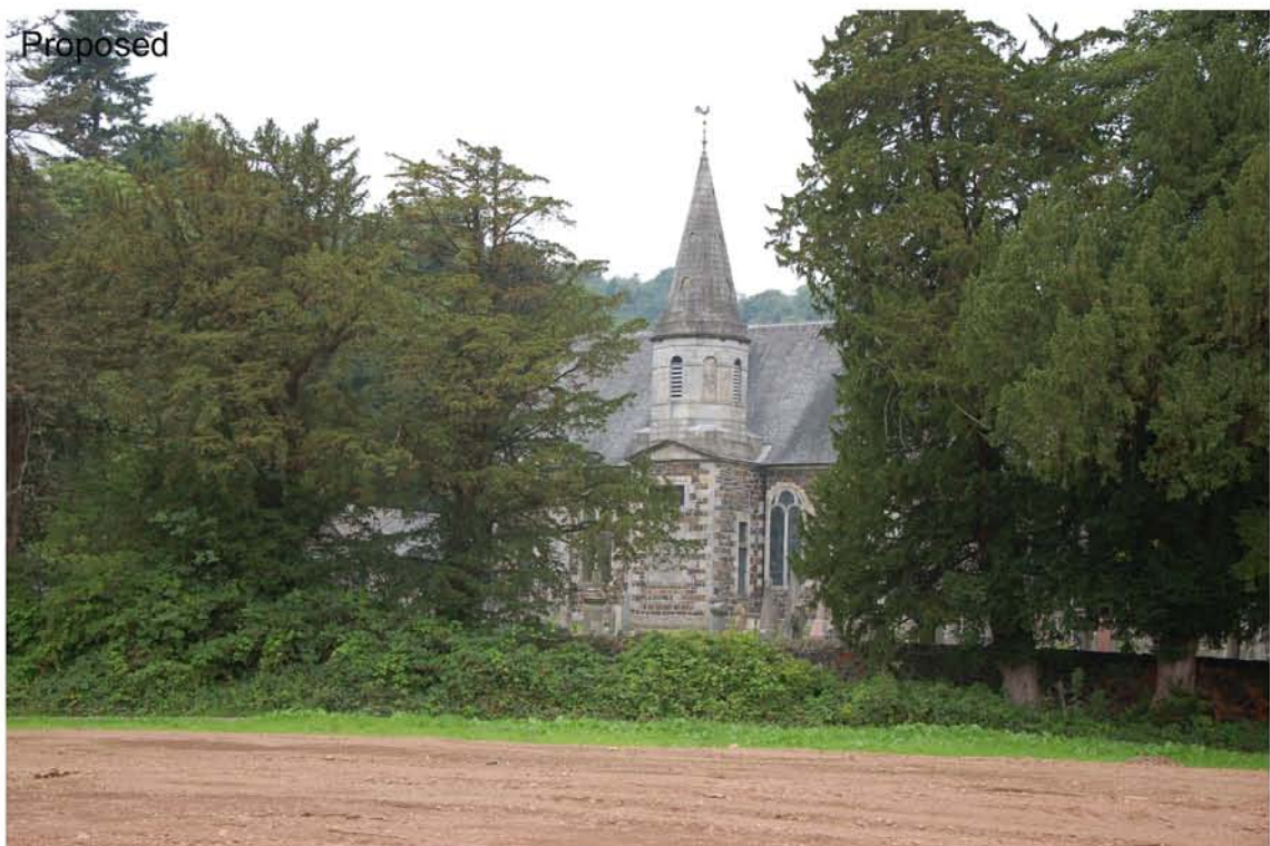
Logie Kirk - view north of the Kirk tower from within the new cemetery area
