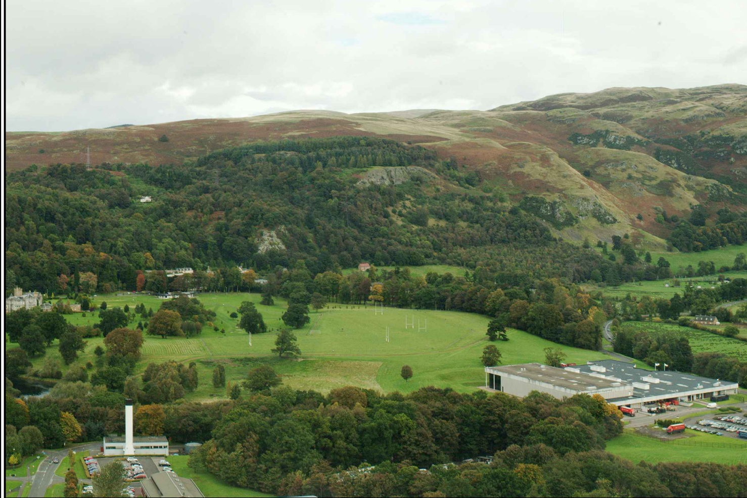
Towers TD202, TD202/1 and TD203 'darkened' to reduce their visibility against the scarp slope
