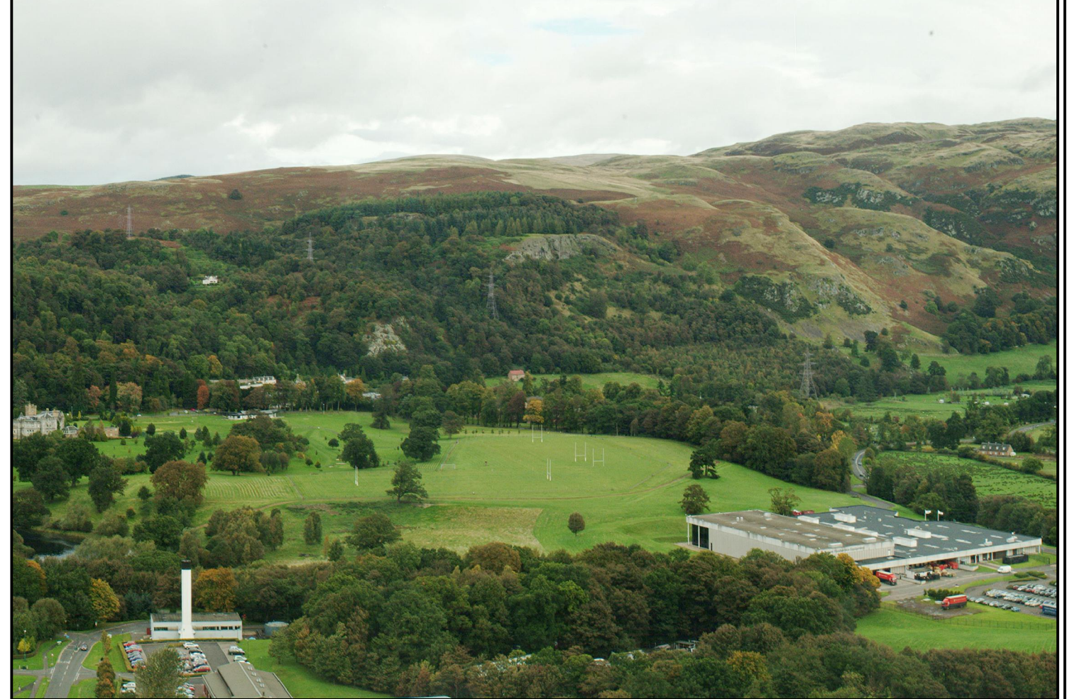
No painting of overhead line towers
