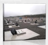
This substation will collect electricity from proposed wind farms and transform it into a suitable voltage to transmit along the overhead line and into the existing electricity network. Work continues to provide the base for the substation and house the mechanical and electrical infrastructure to be installed.
