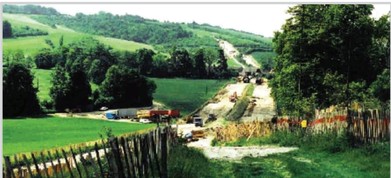
Typical 400kV underground cable construction.
