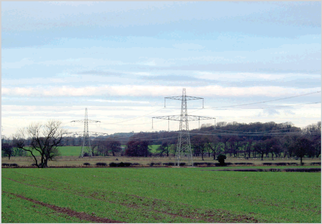
L12 'Low Height' towers near Thirsk, North Yorkshire considered as an alternative.
