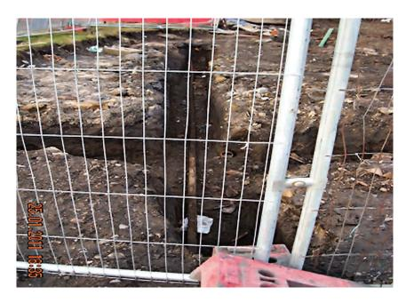
The above image highlights a situation which occurs all too frequently on construction sites. Housing developer proposing to construct a property at the location of a ScottishPower distribution cable.
