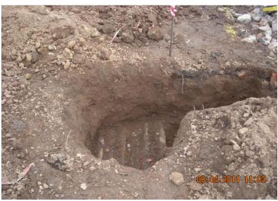
The above image highlights a situation which occurs all too often around the ScottishPower electrical network, 7 high voltage cables had been exposed on a construction site
