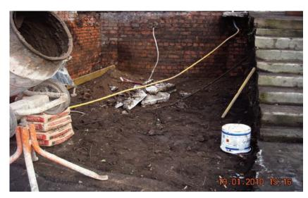
The above image highlights an incident where ground cover was reduced from a small garden to form a car-parking space exposing the low voltage service to the property.
