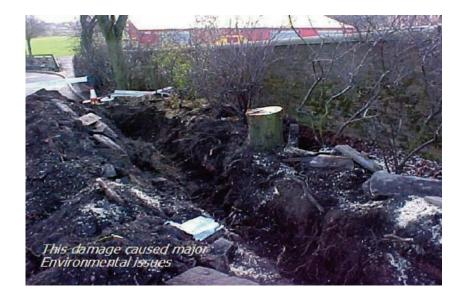
The above Image highlights the consequences of lack of planning when a JCB came into contact with a 33,000 volt oil filled cable.
