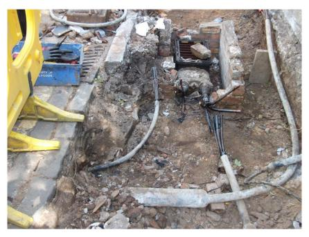
The above image highlights a situation where a low voltage network box requires to be replaced due to a cable fault on the existing electrical network.
