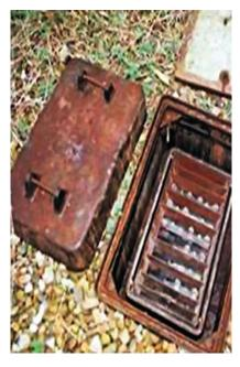
The above images highlight low voltage underground switching boxes (link boxes) protected with a concrete cover.
