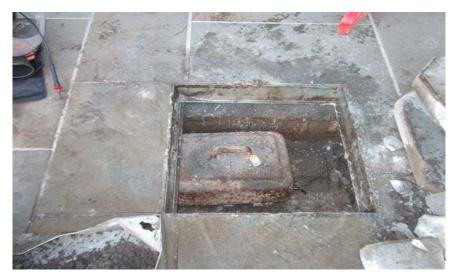
The above image highlights a situation which appears to be on the increase around ScottishPower EnergyNetworks link boxes (underground electrical switching points) the level of streetscape works undertaken by local authorities over recent years has increased.
