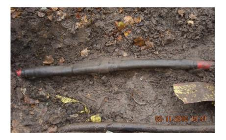
The above image highlights a high voltage cable joint on a Polymeric to Polymeric electrical cable (red cable), operatives undertaking excavations may not have come across this type of joint before, the joint is a sleeve made up of a composition of plastic and rubber (XLPE) and is fit for purpose. Using cables as a step or hand hold to enter or exit excavations is not recommended.
