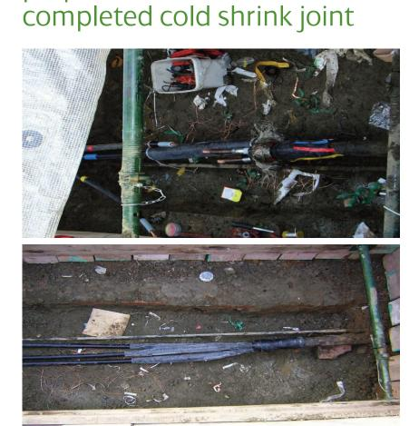
The top image demonstrates a fault on a 33KV cable in the process of being prepared for jointing.
