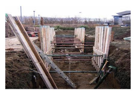
The above image highlights the size of excavations and the correct supporting techniques required to ensure safety at deep excavations.
