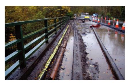
The above image highlights a typical situation were works are being undertaken to re-seal a bridge structure.
