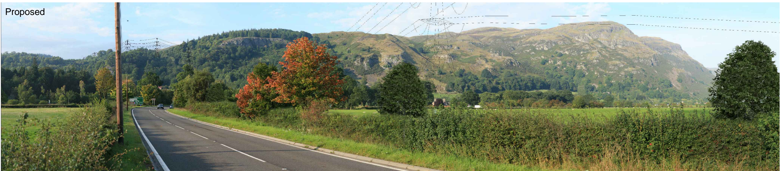
A91, view north and north-east (south of the Logie roundabout), illustrating the proposed planting mitigation measure LV37 and the change in overhead line transmission in this area
