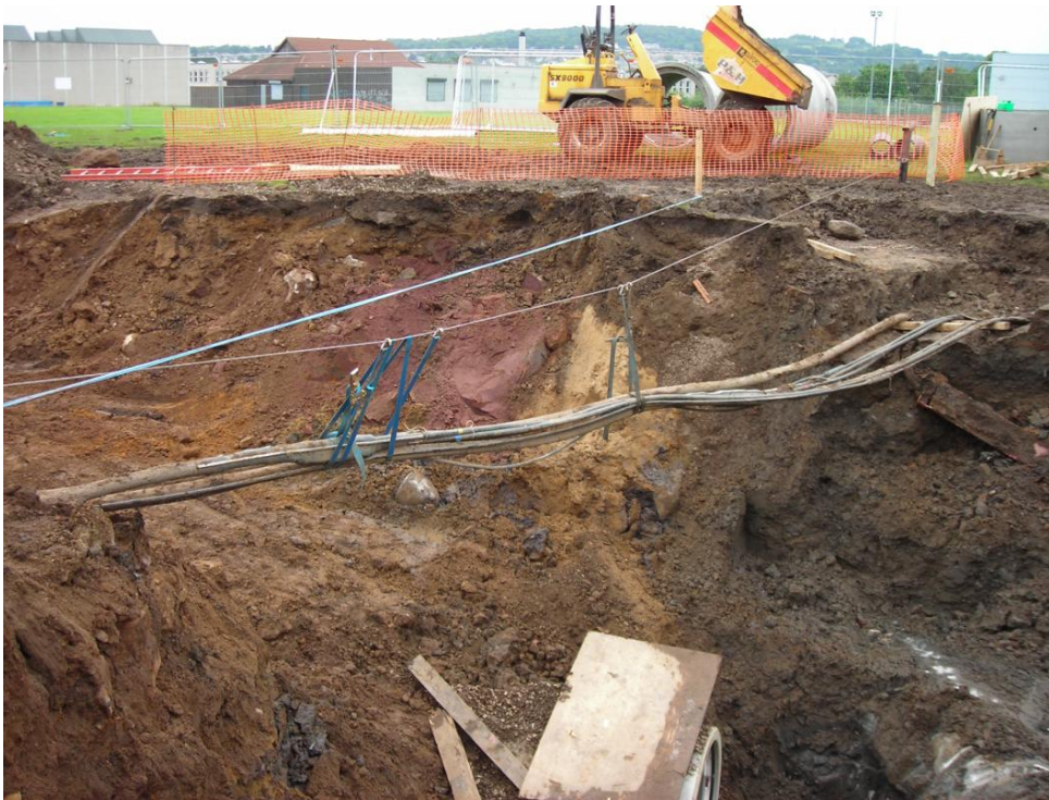
The above image demonstrates how NOT to support electricity cables.
