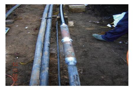
The above image demonstrates a 33kv single core fault repair on the Transmission System, the cable being a 1000mm copper paper insulated lead covered single core.
