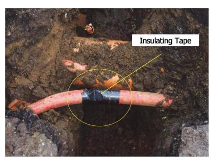
The above image highlights an HV cable damage with a covering of insulating tape applied by an operative.
