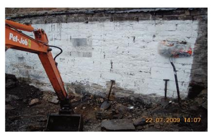
The above image highlights a situation where a garage was in the process of being demolished, exposing a live electrical cable head covered with a plastic bag.
