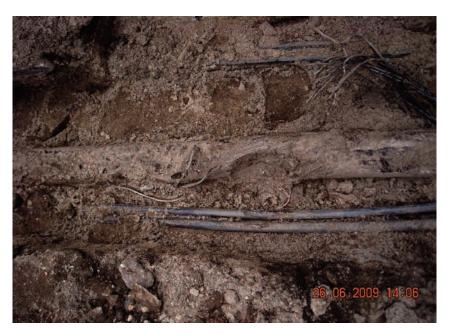
The above image highlights a situation where a 33KV cable was struck while carrying out piling operations.
