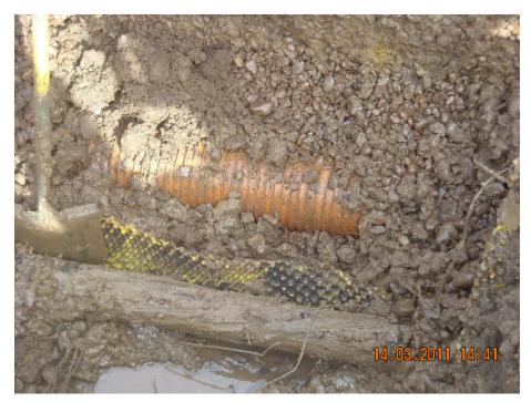
The above image highlights the consequences of lack of separation between ScottishPowers 33KV wired armoured cable and the newly installed field drain
