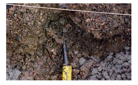
The above image is an example of poor working practice, a gas pipe being used as a duct for an electricity service cable.
