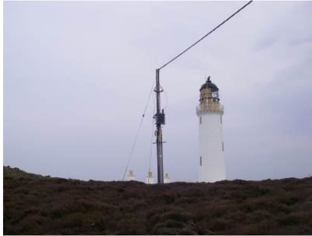
Figure 28 – Ericsson Cable (Mull of Galloway Lighthouse)
