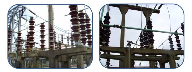
The disconnectors and the civil structures which support them have gradually deteriorated over time. The ongoing costs associated with the repair and maintenance is high, and the condition of this asset has added to the overall justification for 132kV plant replacement. Full site condition details are contained within our 132kV survey reports.
