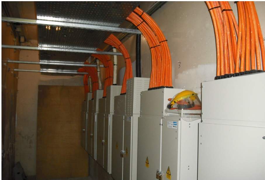
Figure 5 – Example of modernised RLM system
