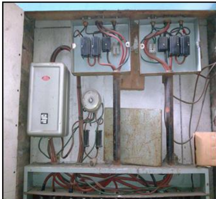
Figure 4 - Example of a typical HI5 RLM system
