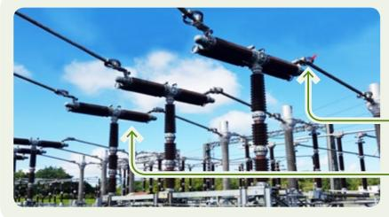
Air Insulated Switchgear (AIS) uses air to insulate the high voltage connections from earth
