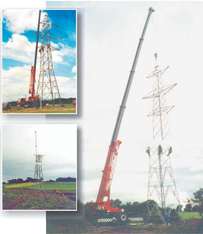
Construction of typical L4 tower
