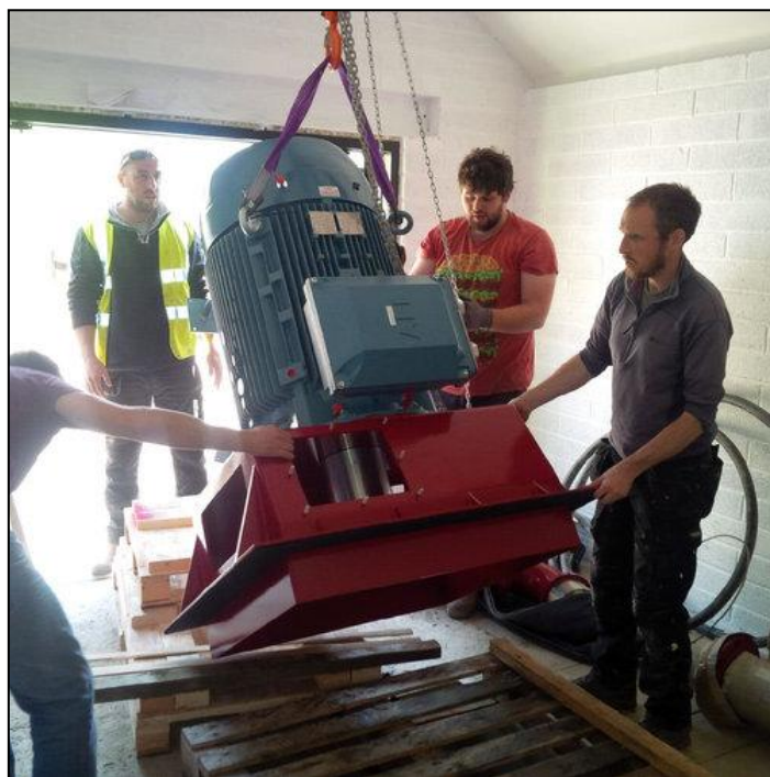
Figure 15 Hydro generator being installed at Hydro Ogwen, near Bethesda
