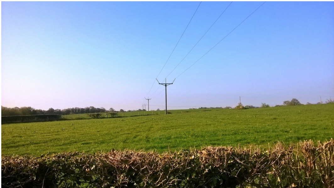
Figure 2.2 Photograph of an existing 132kV ‘Trident’ overhead line in North Wales.
