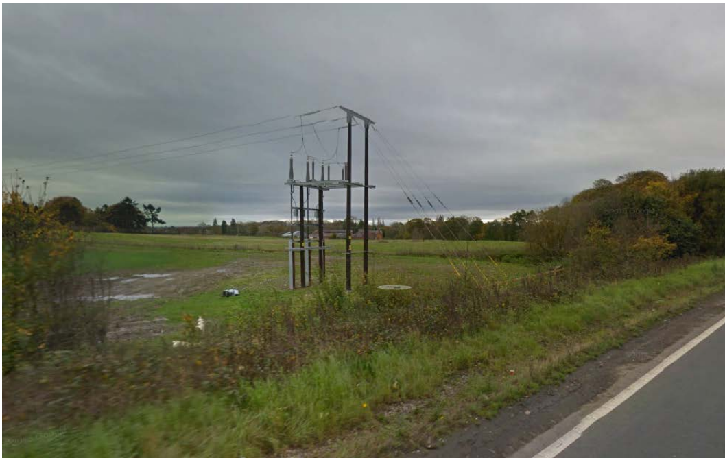
Figure 4. Photograph of a 132kV wood pole Trident overhead line termination.
