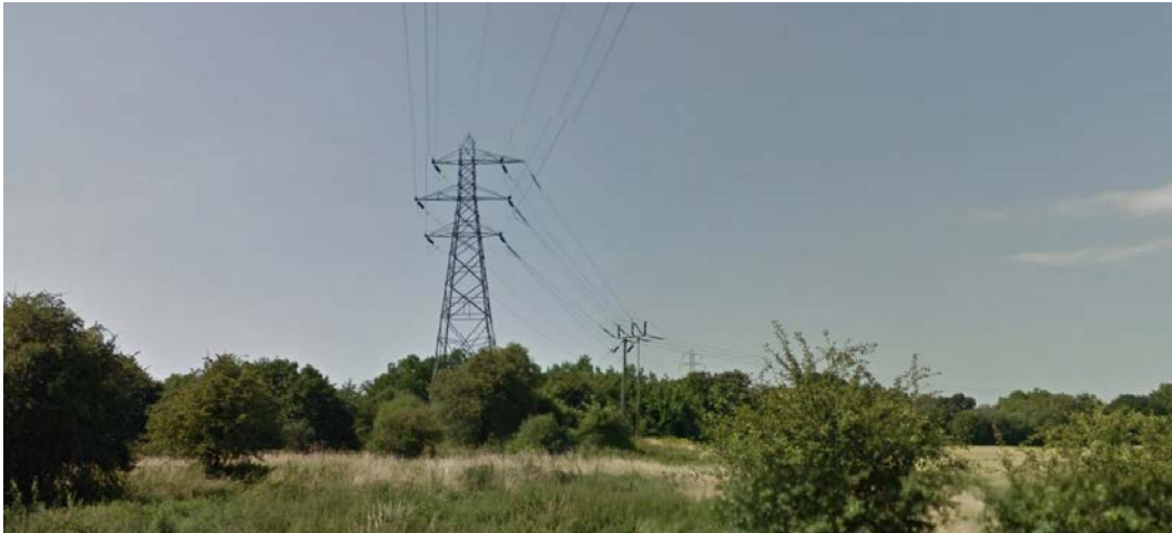
Figure 3. Photograph of a tee-off arrangement from a 132kV tower line to a 132kV wood pole line.
