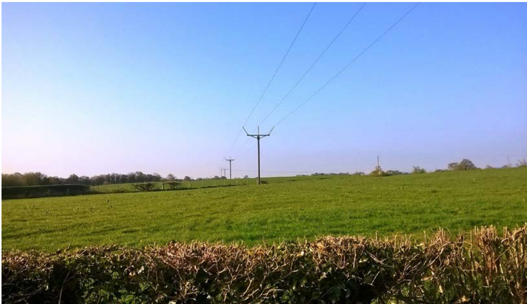
Figure 2. Photograph of a 132kV wood pole Trident overhead line.
