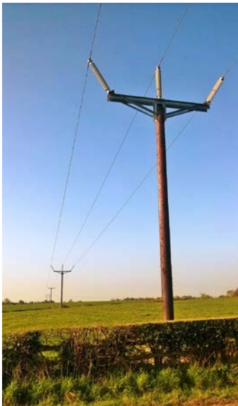
Figure 5 (left). Typical 132kV Trident wood pole overhead line.
