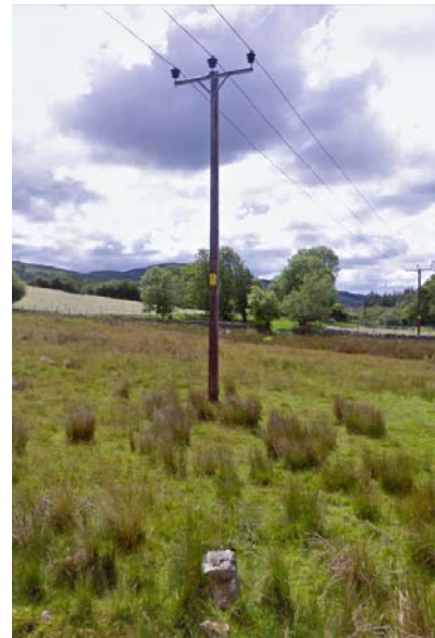
Figure 6 (right). Typical 33kV wood pole overhead line.
