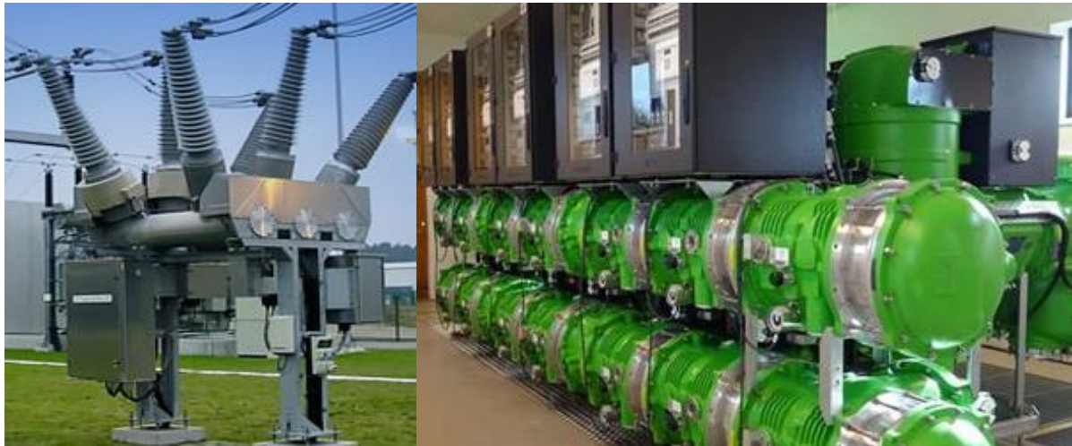
Figure 32: “Dead tank” Circuit Breaker (~36kg SF 6 ) & 132kV GIS Alt Gas Switchboard (G 3 )
