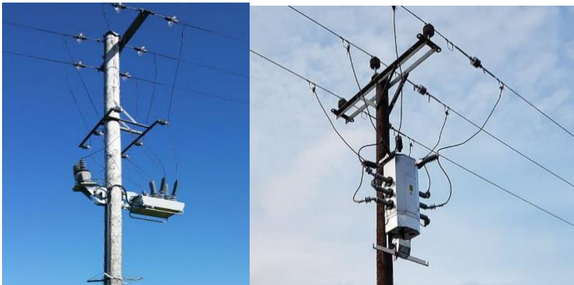
Figure 36: 11kV NOJA OSM 15 Recloser (solid/vacuum) & 11kV ENTISO Auguste SF 6 Switch (1.9kg SF 6 )
