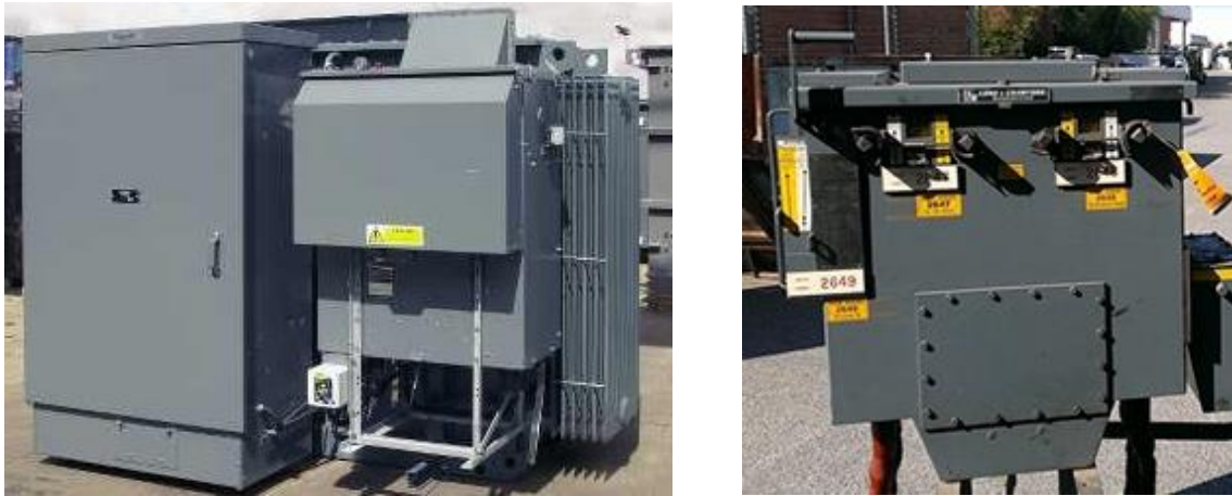
Figure 35: 11kV Packaged Substation, RMU (0.5kg SF 6 ) & Legacy 11kV Oil Filled Ring Main Unit (Nil)
