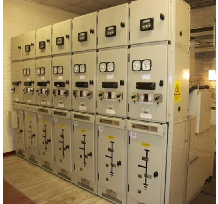
Figure 34: 11kV Primary Switchgear Vacuum retrofit (Nil) & 11kV SF 6 Primary Switchgear (~0.5kg SF 6 )
