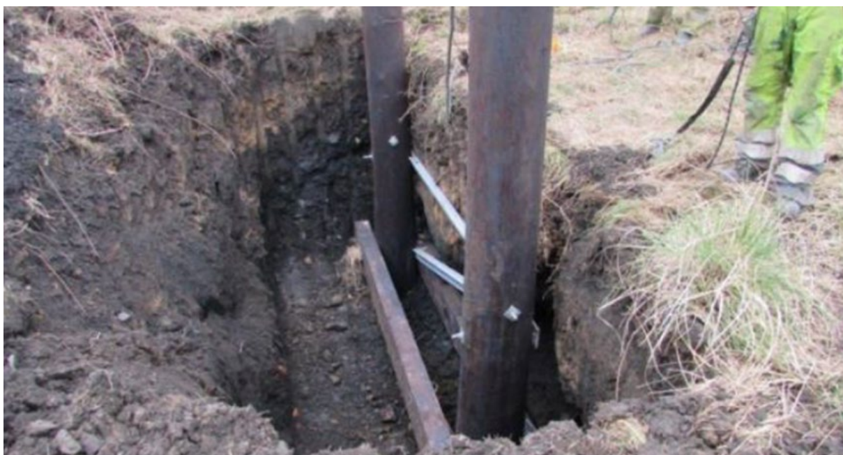
Photo 5: Wood Pole Foundation (Intermediate H-pole)
