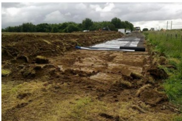
Photo 7: Temporary Composite Roadway Panels
