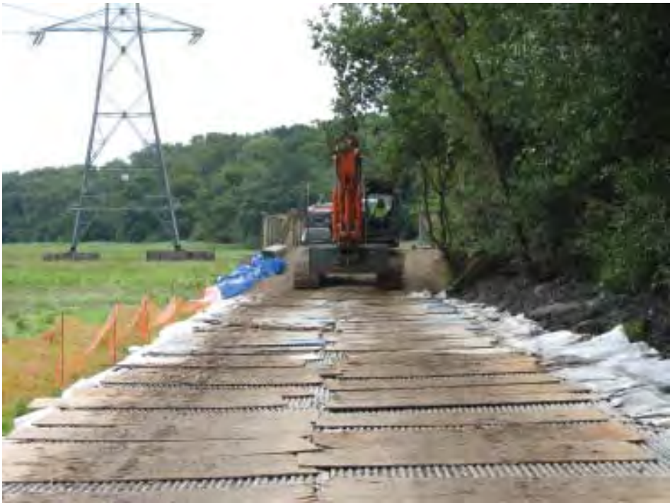
Figure 5.19 - Floating tracks/steel matting/Low pressure access track
