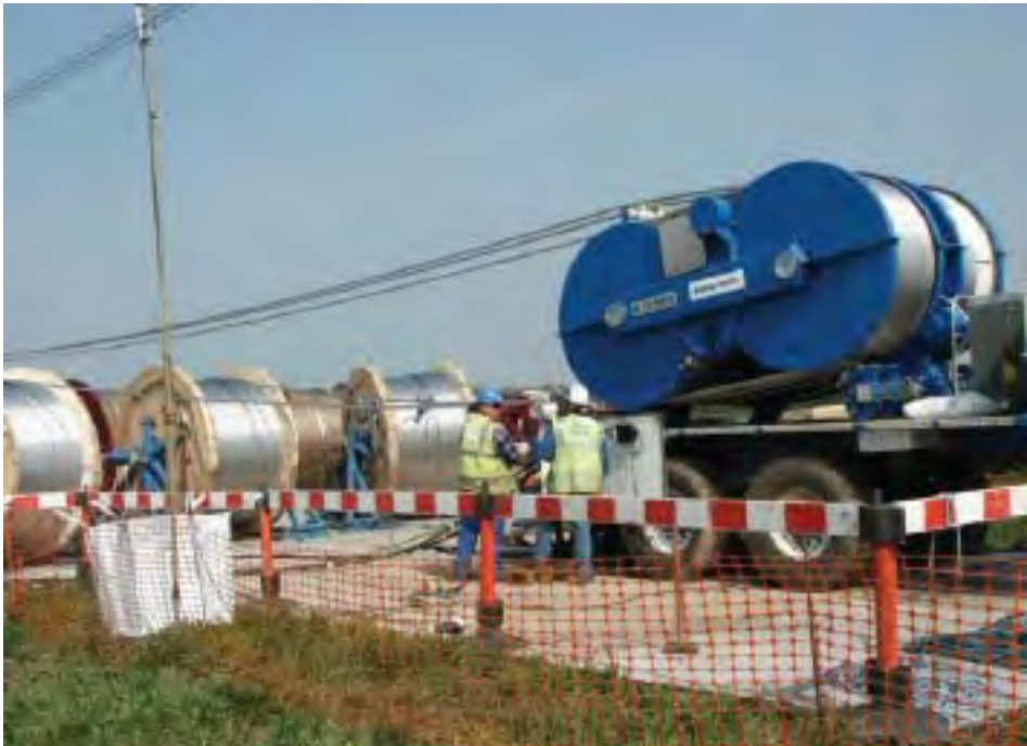
Figure 5.24 - Conductor stringing, L7 Towers
